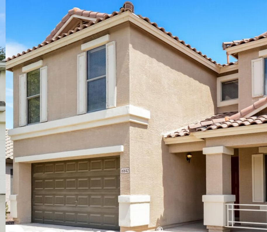
Progress Residential Energy Saver Home — Phoenix, Arizona
